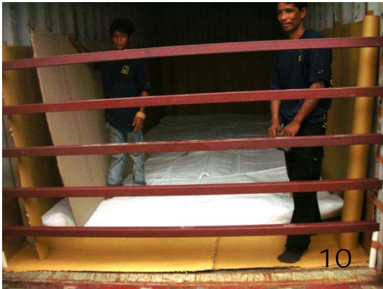
Pictured Metal bar for bottom discharge flexi bag placement. For top discharge bags, the bottom bar should sit 2 inches from floor, or on bracket at groove.
